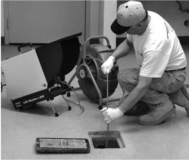
Figure 28 – Proper Cable Push
